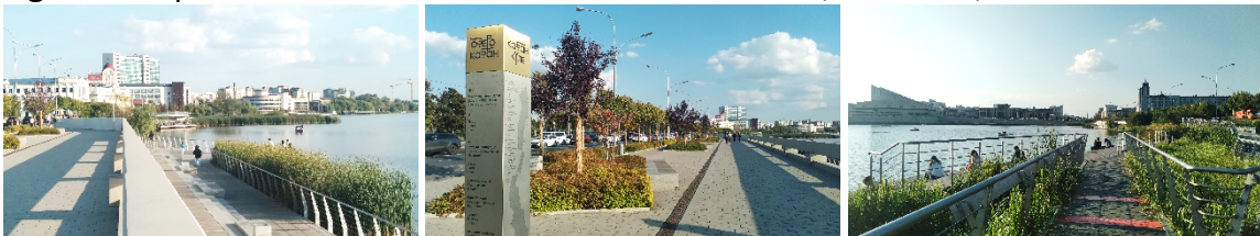
Figure 9. Improvement Kaban lake embankment in Kazan, Tatarstan, Russia
